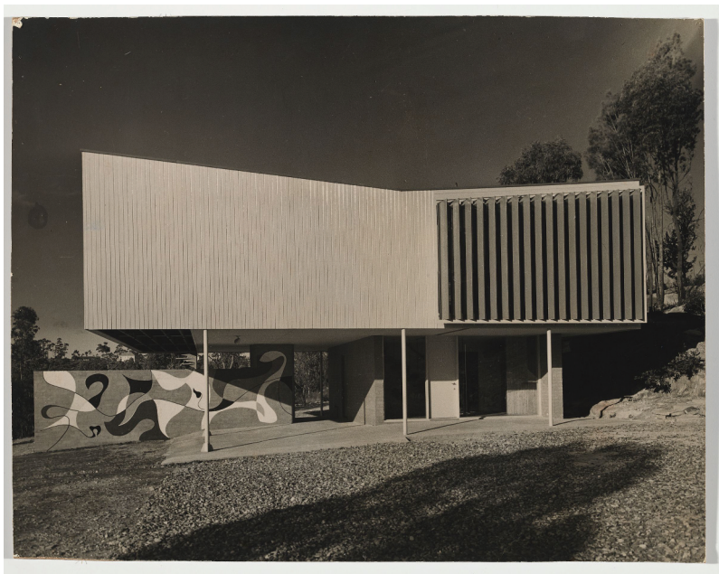
Figure 4. Adjustable louvres and mural by Harry Seidler at the Marcus Seidler House, Wahroonga, New South Wales, 1949-51. Architect Harry Seidler. Photograph, 1953 by Marcell Seidler. Source: National Gallery of Australia (NGA2001.250). Copyright Penelope Seidler.
